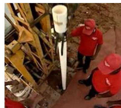
Lower the pump by screwing in the pipe sections.
