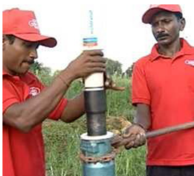
Screw in the first PYD pipe section.
