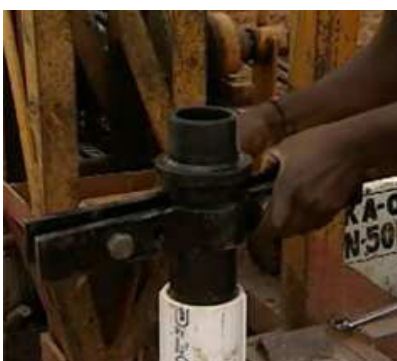
Attach the suspension system and let it rest in the well.
