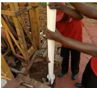
Insert lower adaptor at pump outlet.
