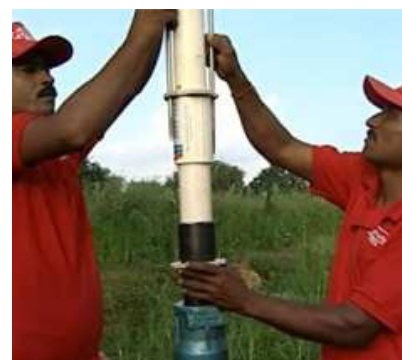
Attachment of the motor guard to the lower adapter.
