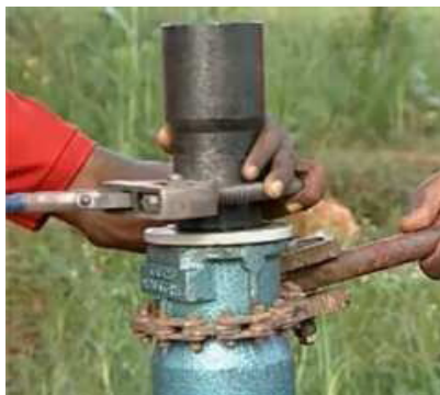
Thread lower adaptor to pump outlet.
